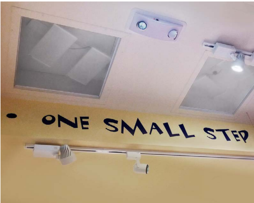
A Build-a-Bear Workshop using directional audio speakers to enhance its interactive workstations.
